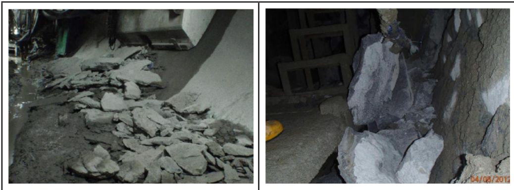
Figure 4. Rock burst in TBM 2 at Ch. 24610
