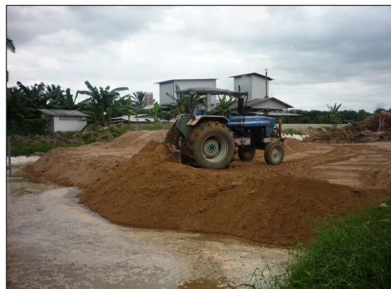
Figure 2. The fill and compaction process were done on the surface of marine clay soil
