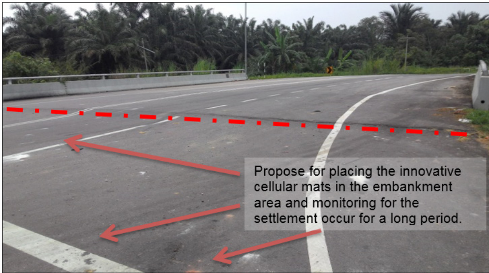
Figure 11. The field settlement design/mode (propose) shown in embankment area jointed with concrete bridge located at Parit Yaani, Batu Pahat, Johor.
