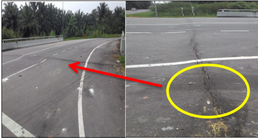
Figure 4. The current situation of site observation (taken on October 22, 2015) with the increment angle of the slant/edge of the embankment approaching to the Parit Yaani's bridge
