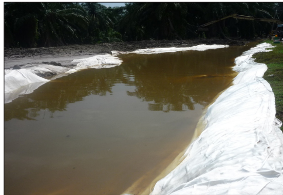
Figure 1. The marine clay deposited along Parit Yaani's river covered with geotextile in 2010
